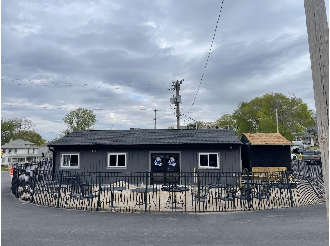
Figure 1: Existing patio where the open pergola is proposed to be located.
