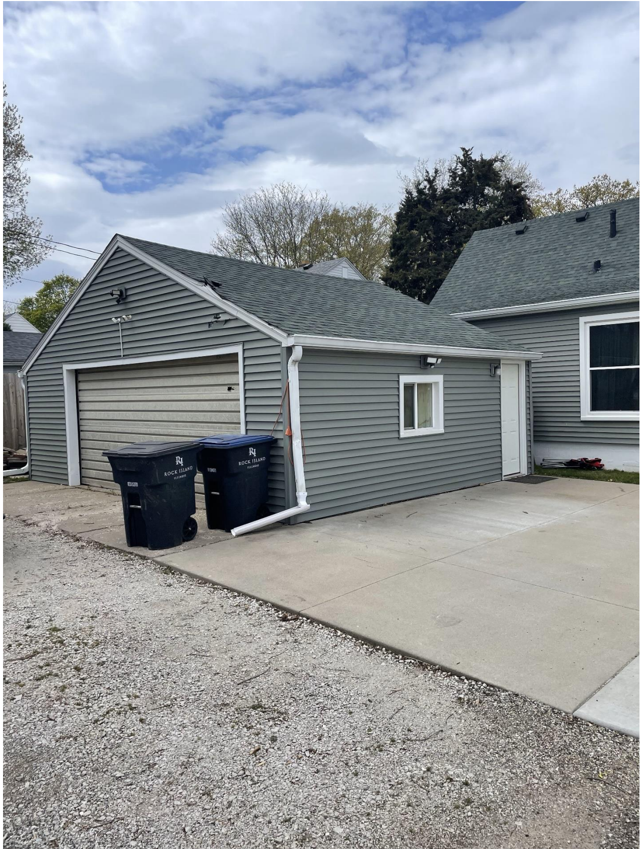
Figure 1: View of existing garage at 2140 23rd Avenue.
