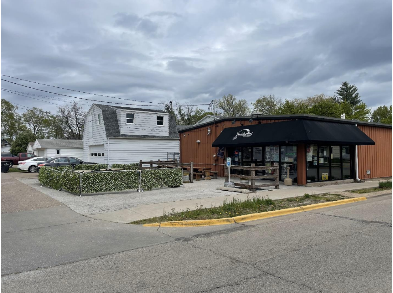
Figure 1: View of temporary patio setup on the property.
