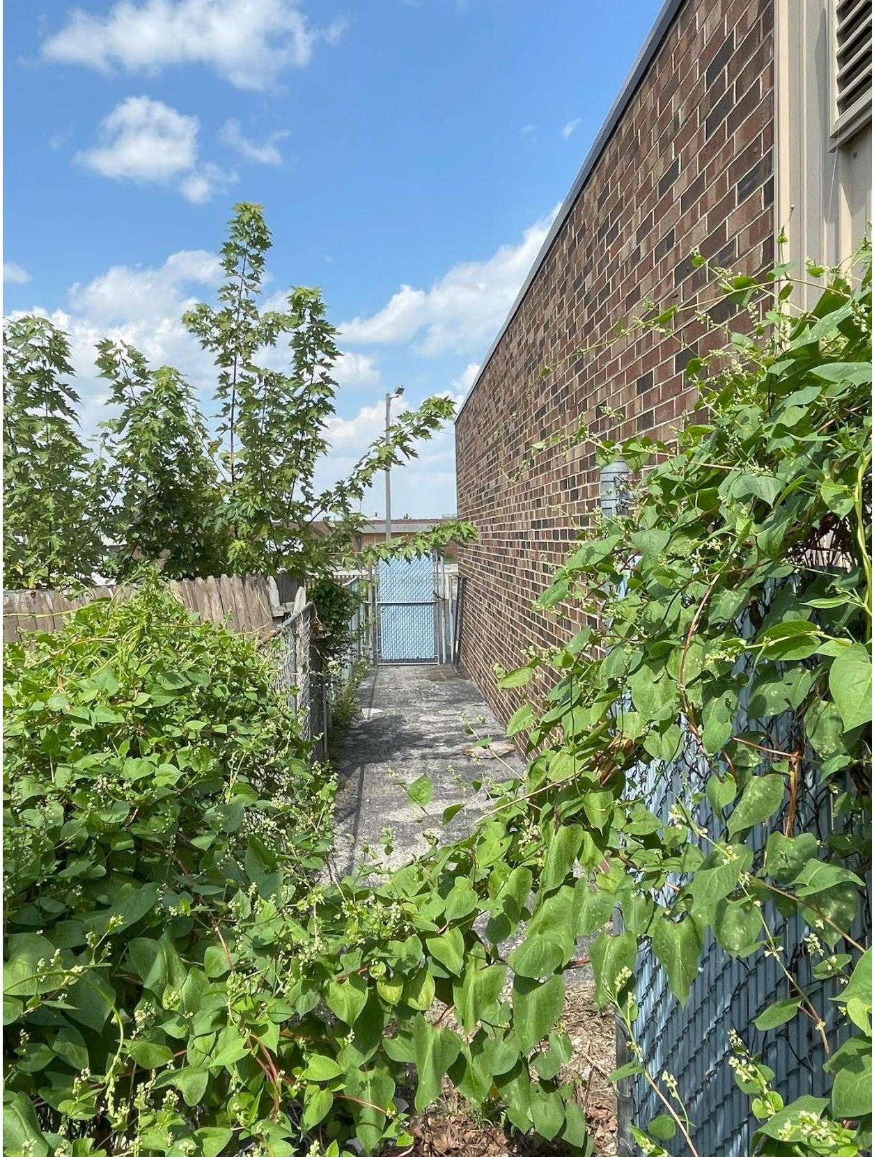
Figure 2: Photo of proposed storage area looking north towards 7th Avenue.
