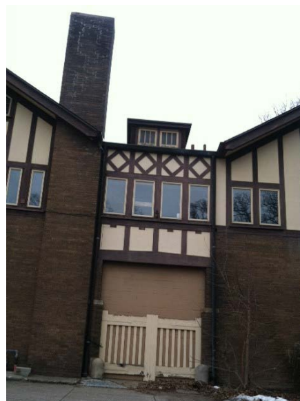
Center East Façade (Original Entrance) With Original Gate
