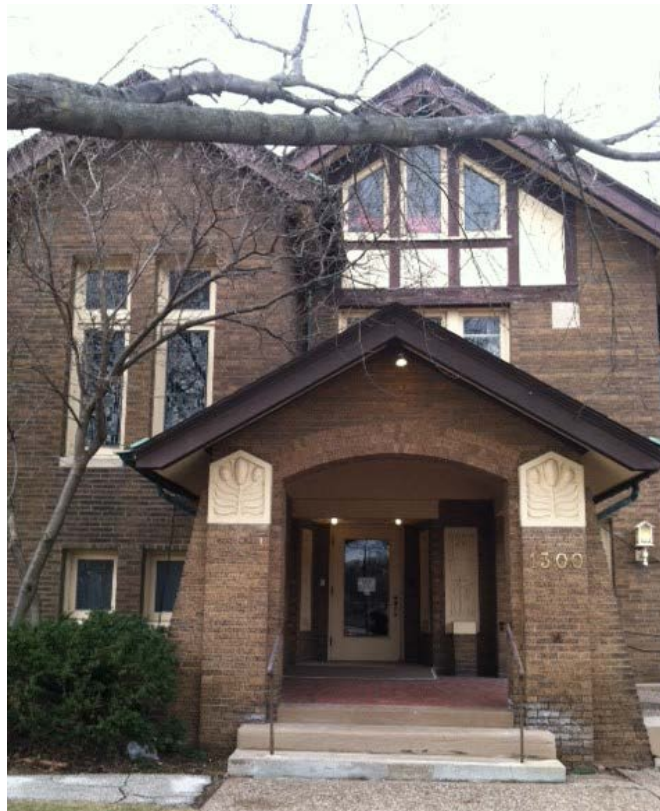
Front Façade Center (faces southeast)
