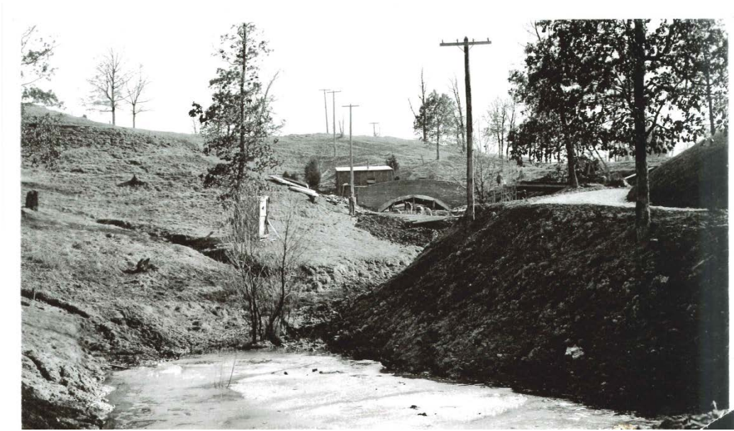
View of the Bridge and one of the Ponds During Construction ca. 1911
